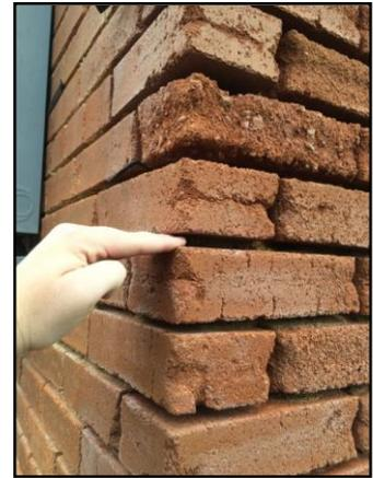
*The mortar on this brick wall needs to be replaced to prevent collapse.*
